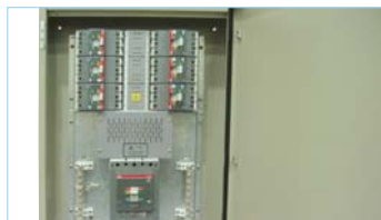
MCCB Pan Assembly Panel Board
