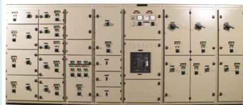
Chiller Control Panel/Main Air Conditioning Switchboard
