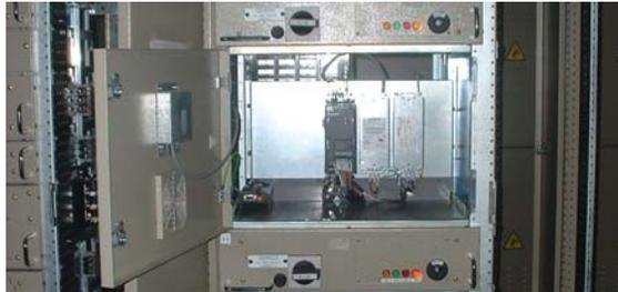
The complete modular system allows maximum freedom when designing Motor Control Centre (MCC). The physical dimensions of each compartment can be varied in width, height and depth to accommodate the various space requirements for different starter types:
